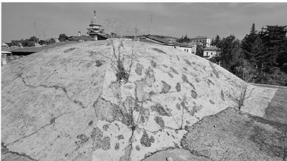
Picture 8 Concrete slab outer view
