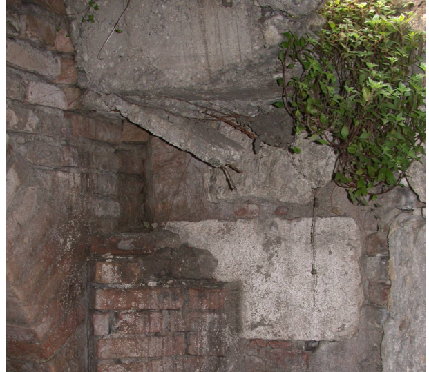
Picture 10 Concrete slab interior view
