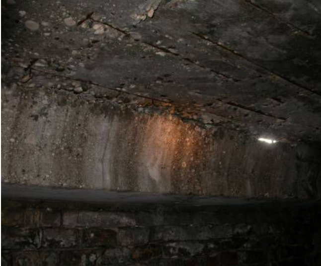
Picture 9 Concrete slab interior view
