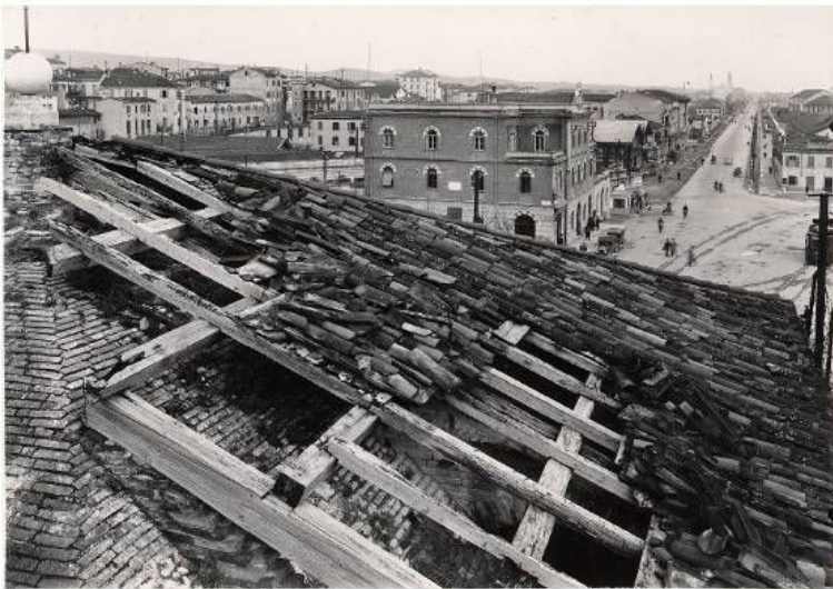
Picture 5 Other picture of 1930 roof demolition
