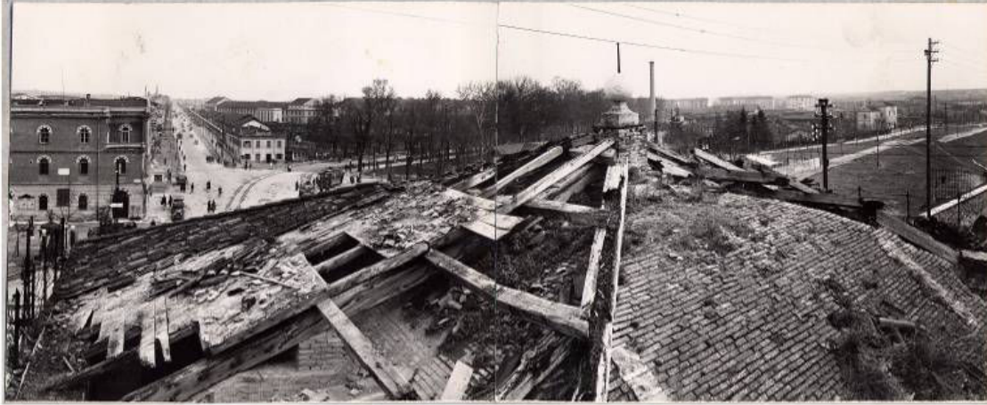
Picture 4 Demolition of timber roof in 1920-1930
